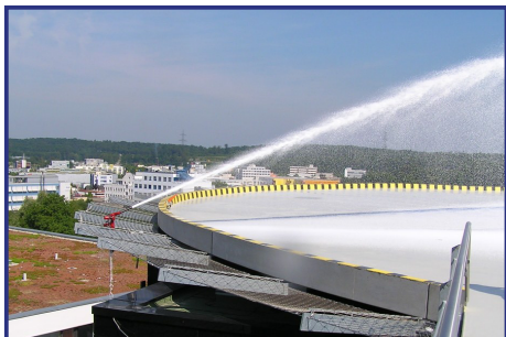
ONE SEVEN® HELI PAD INSTALLATION
