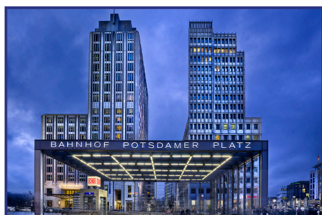
CABLE DUCT RAILROAD STATION POTSDAMER PLATZ, BERLIN
